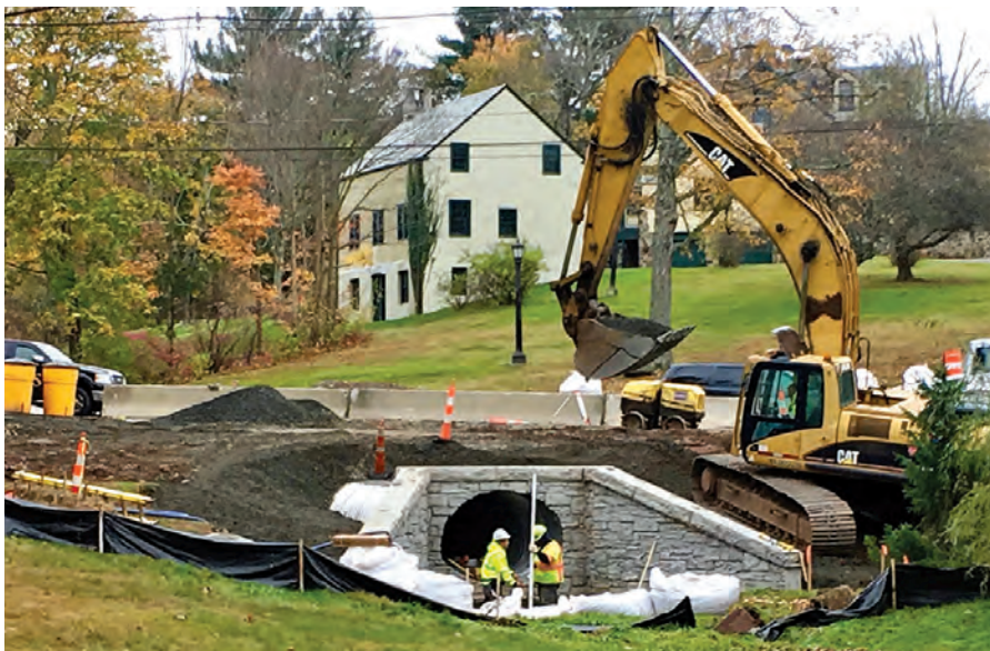
The nearly finished culvert at Boulder Brook
